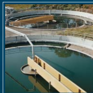
Waste Water Treatment Plant
